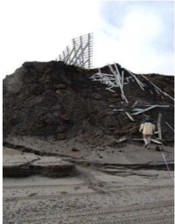
Figure 8: Shoreline Erosion (Source: Army Corps)
