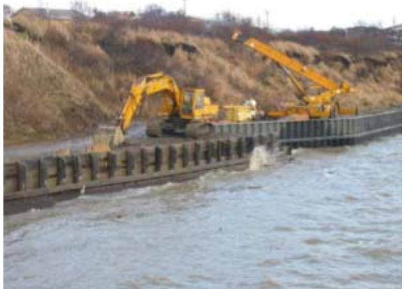
Figure 7 Corps Shore protection at Snag Point (Source: Army Corps)
