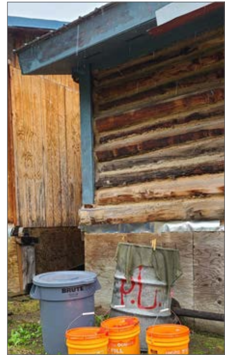
Catching rainwater at a house in Koyukuk. Photo Credit: Department of Commerce, Community and Economic Development; Division of Community and Regional Affairs' Community Photo Library.
