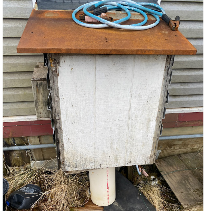
New Stuyahok Arctic Box Repairs
