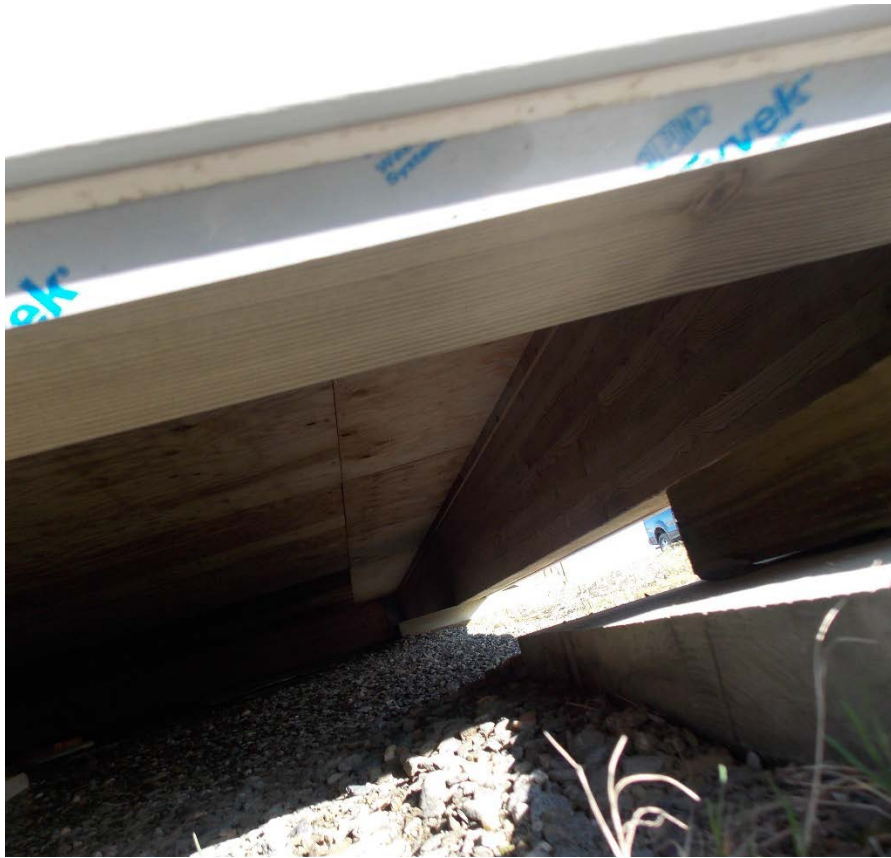
Exterior subfloor under the office appears to be in excellent condition.
