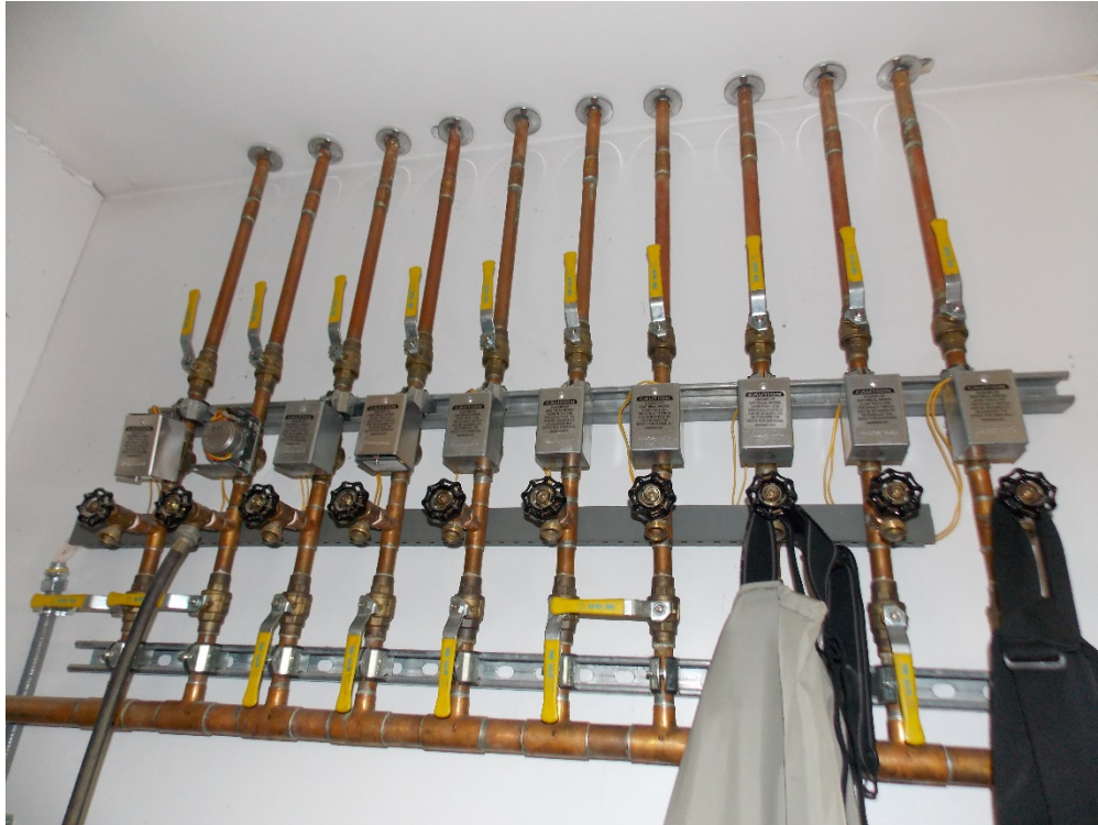
Plumbing was not insulated in the boiler room. Installing foam insulation around the copper pipe would prevent heat loss through the hot water lines. Insulation would also prevent condensation build-up on the cold water pipes.
