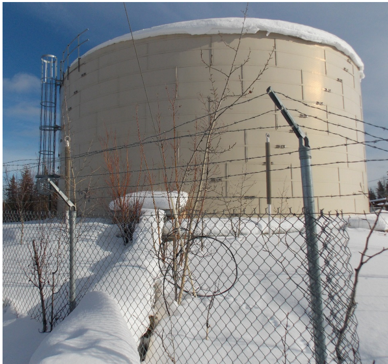
Figure 4: Water storage utilidor and tank.
