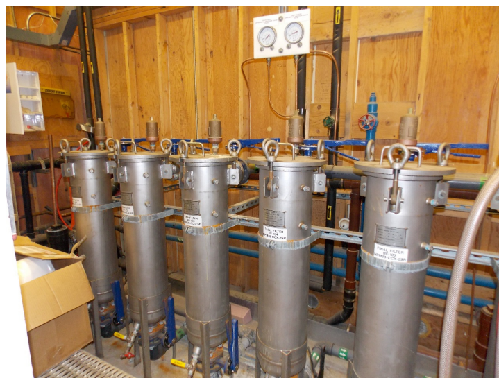
Figure 3: The water treatment plant bag filtration system.
