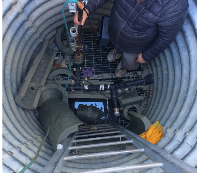
Figures 2a. (left): Venetie pump house. Figure 2b. (right): Venetie sump. The lower line from the pump house (coming in from the left) connects to the upper line (going out to the right), which runs to the water treatment plant. The stub out in the center of the photo is the drain port.
