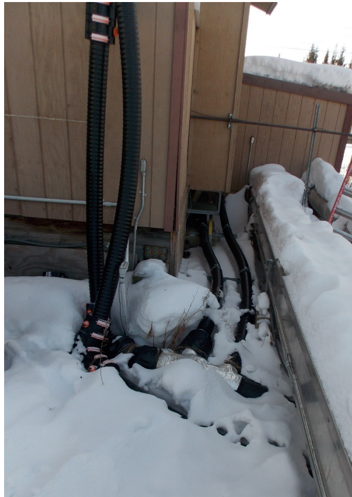
Figure 7: Exterior heat recovery transmission line (black flexible pipe). The piping running parallel to the water storage tank utility is a node to the clinic.
