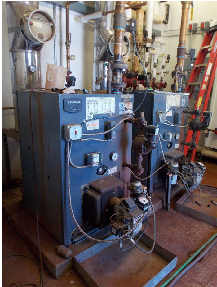
Figure 5: Weil-McLain 480 Commercial boilers.
