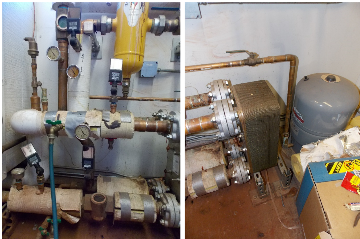
Figure 6: Heat recovery system (left) and heat exchanger (right) in the water treatment plant boiler room.
