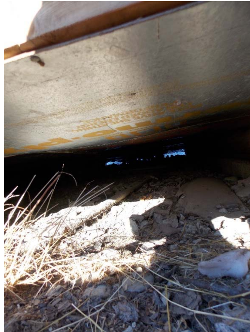
The exterior roof and subflooring are not well sealed. The fiberglass batt is likely to be damaged from exposure to the elements and moisture.
