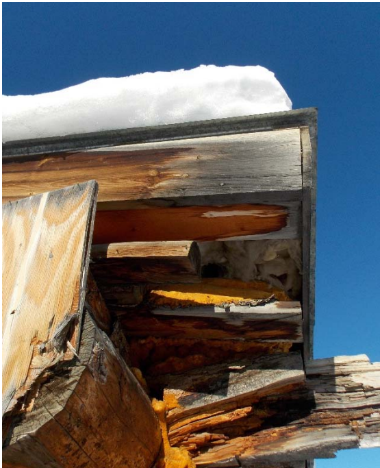
The exterior roof and subflooring are not well sealed. The fiberglass batt is likely to be damaged from exposure to the elements and moisture.
