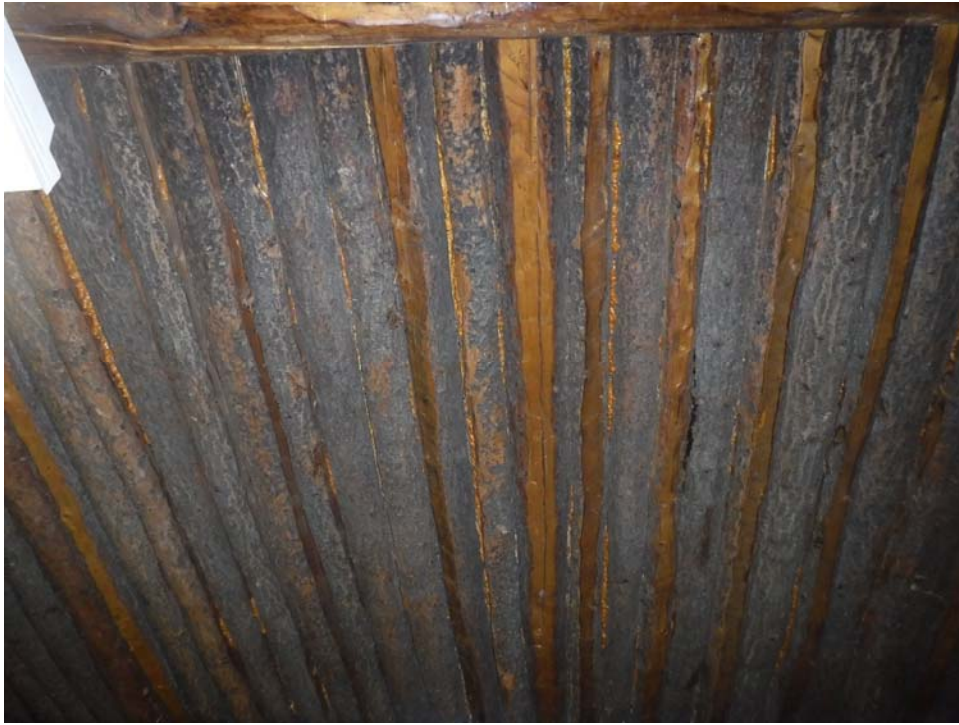
Council Office interior ceiling construction.
