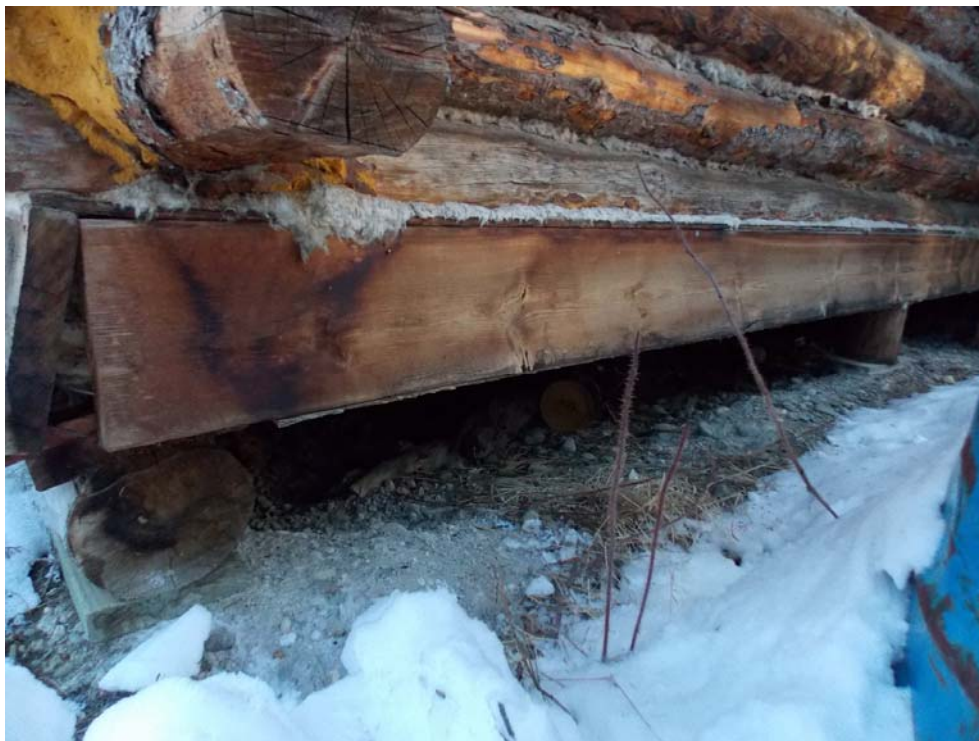
Council Office's flooring exterior.
