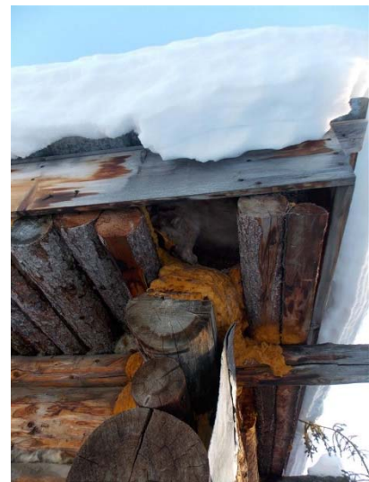
Typical roofing structure in Venetie.
