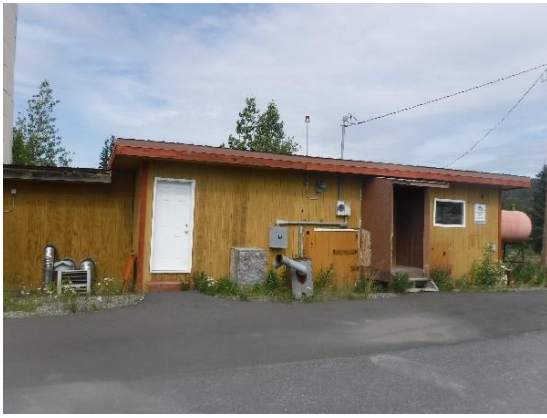
Figure 11: Old Water Treatment Plant
