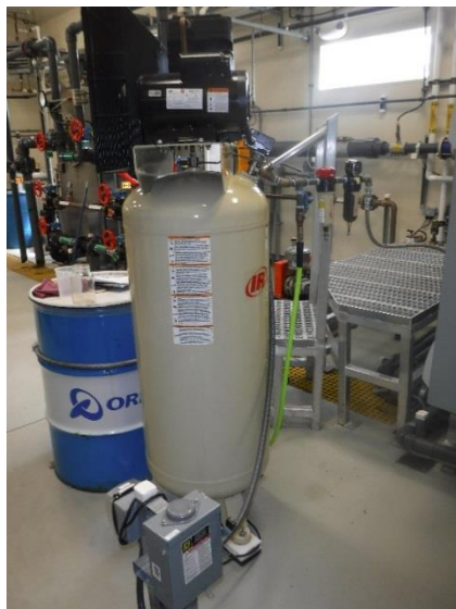
Figure 18: MIEX Air Compressor
