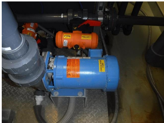
Figure 17: MIEX Circulation Pump
