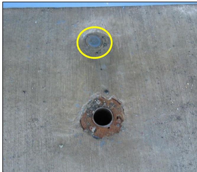
Figure 1.6: Honeywell Ice Sensor for the watering point drain heat trace.
