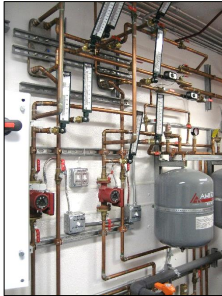
Figure 1.5: Water Building water and sewer glycol heat trace controls and heat exchangers.
