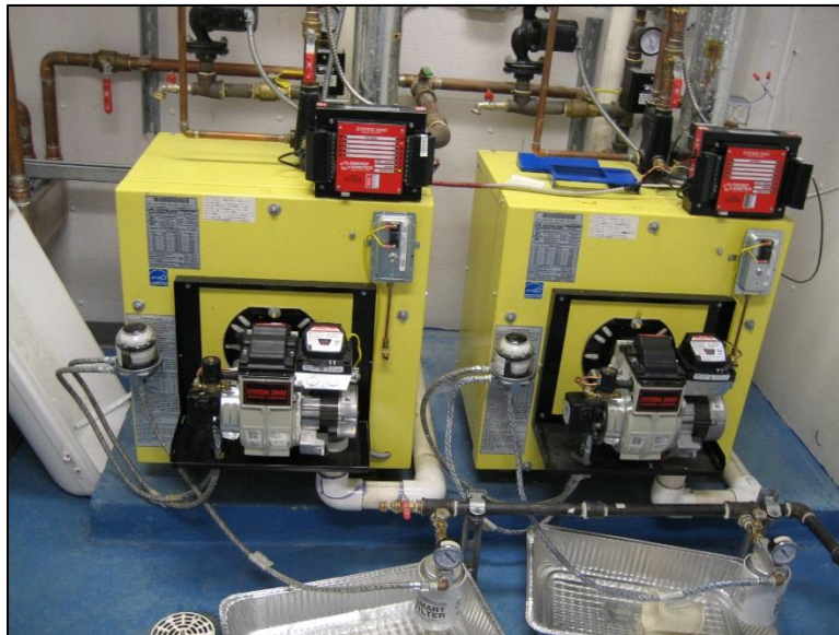
Figure 1.2: Chistochina Water Building boilers.
