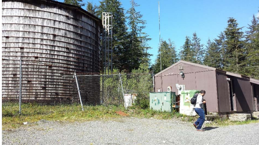
Figure 12: Wood Stave Tank (left). Yakutat Water Treatment Plant exterior (right).
