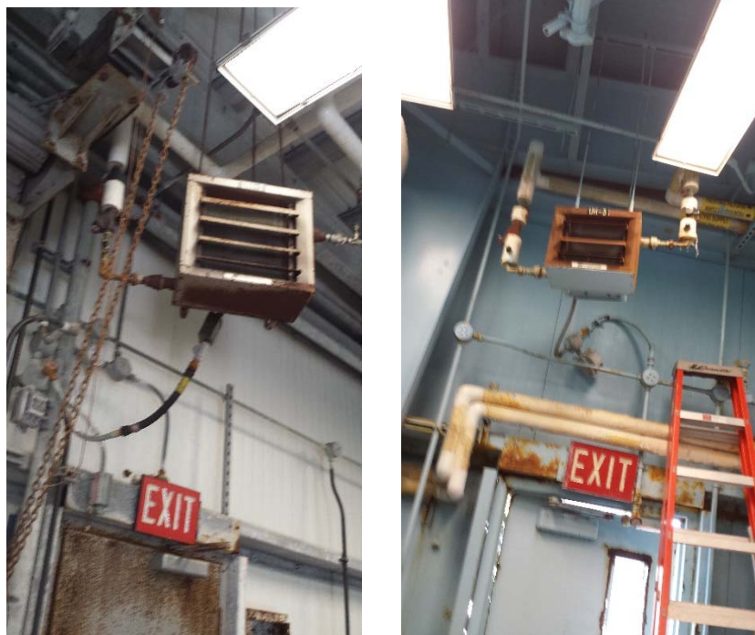
Figure 17: Wastewater Treatment Plant unit heaters.
