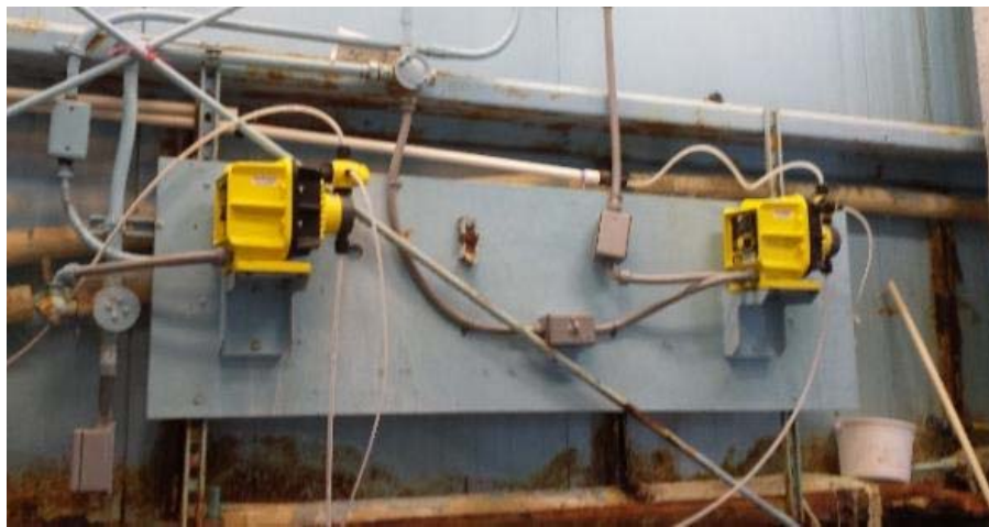
Figure 20: Chlorine disinfection pumps.
