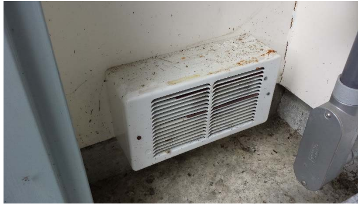
Figure 16: YTT Lift Station Control Room electric heater.
