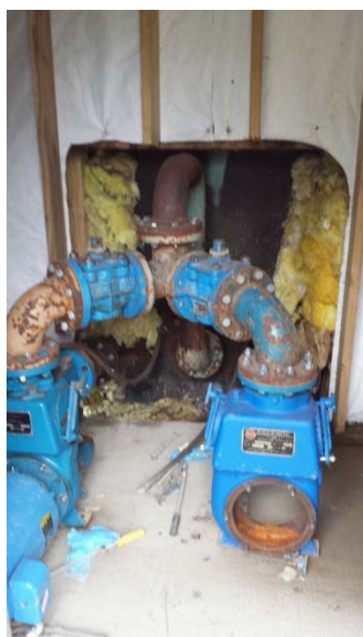
Figure 24: Village Lift Station pumps.
