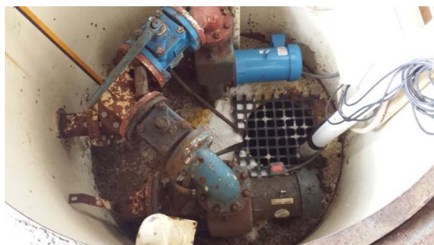
Figure 22: Fish Plant Lift Station pumps.
