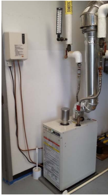
Figure 12: Toyotomi OM-148 hot water heater.
