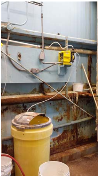
Chlorine disinfectant pump.
