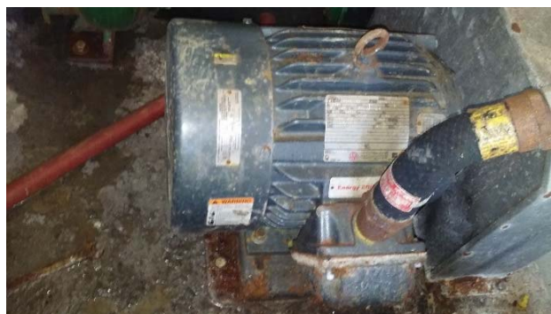
Figure 23: YTT Lift Station pump motor.
