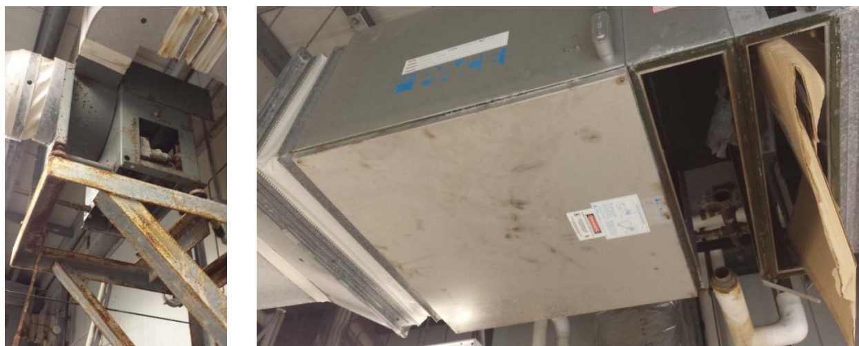
Figure 18: Exhaust Fan above grit screens (left). The PACE Air Handling unit and previous heat-add pipe (right).
