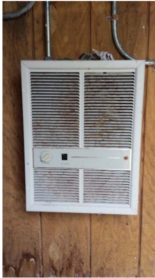
Figure 14: Lagoon Lift Station electric heater.
