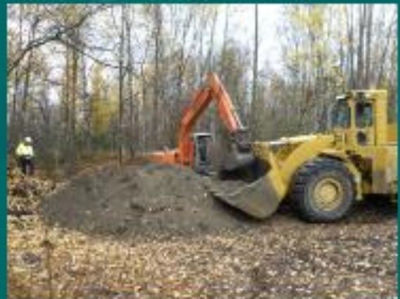
206 tons of contaminated soil were removed for disposal.
