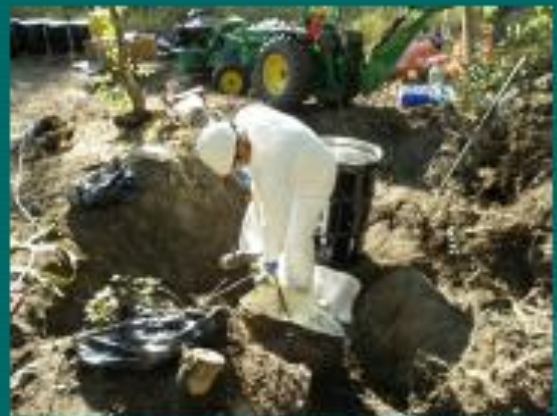
Some drums were banged up. Contents were assessed and condensed for containment.
