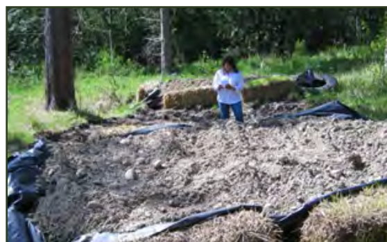
Onsite land farming treatment of heavy oil/SVOC contaminated soil.
