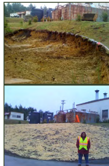
Interim Remedial Action at AOC D (Transformer Spill Site)
