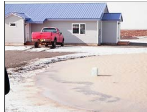
Warm winter temperatures cause localized flooding on top of household septic fields.
