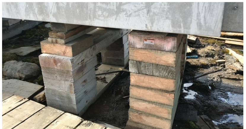
Above is an example of lumber supports that stabilize utilidors during permafrost shifting. The lumber supports will be replaced with helical piles (left,) which are metal pipes driven into the ground. Helical piles will eliminate the need for having to redo the lumber supports, which tends to rot and break down over time.
