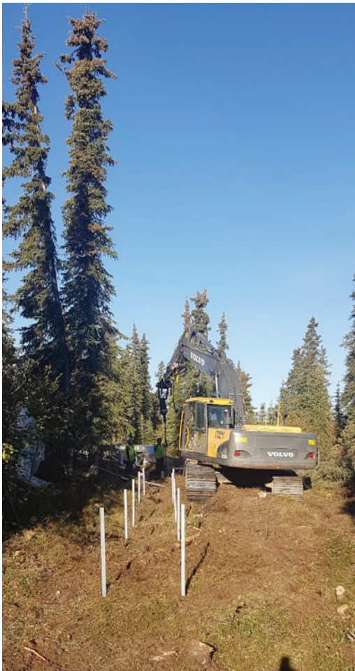
Above is an example of lumber supports that stabilize utilidors during permafrost shifting. The lumber supports will be replaced with helical piles (left,) which are metal pipes driven into the ground. Helical piles will eliminate the need for having to redo the lumber supports, which tends to rot and break down over time.
