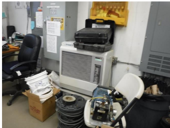
Figure 3: Toyo Stove in the Office Area
