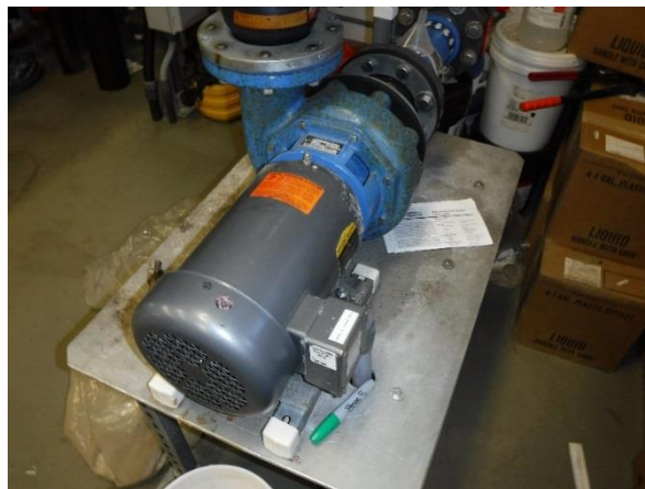
Figure 6: Backwash Pump
