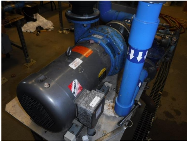
Figure 7: High Capacity Pump
