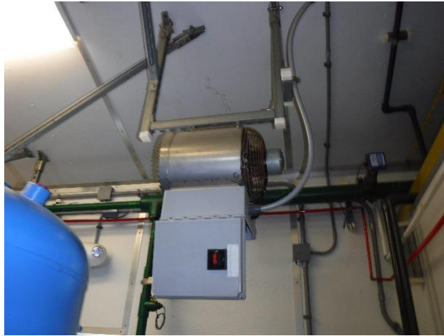
Figure 4: Process Room Electric Heater
