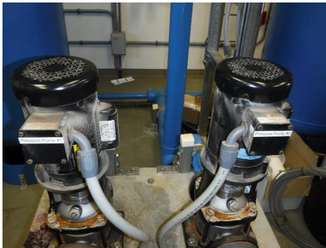
Figure 8: Indian Creek Pressure Pumps
