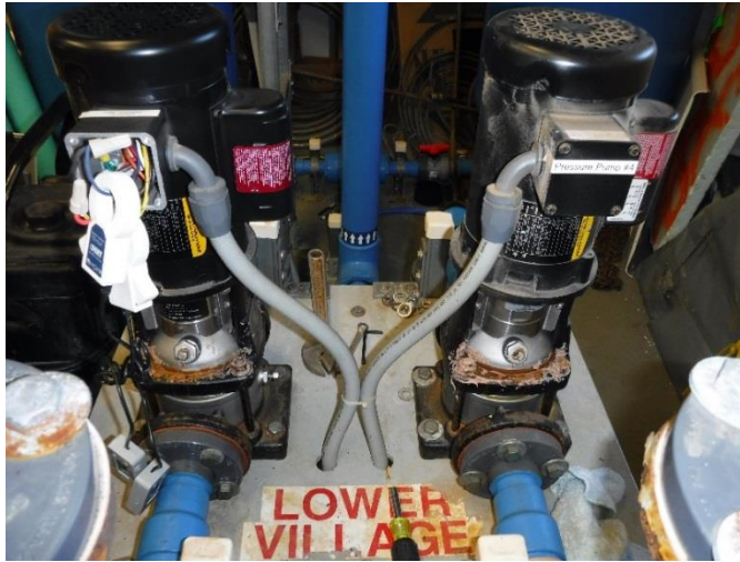
Figure 9: Lower Village Pressure Pumps
