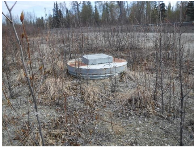
Figure 1: Tyonek Water Treatment Plant Well 1
