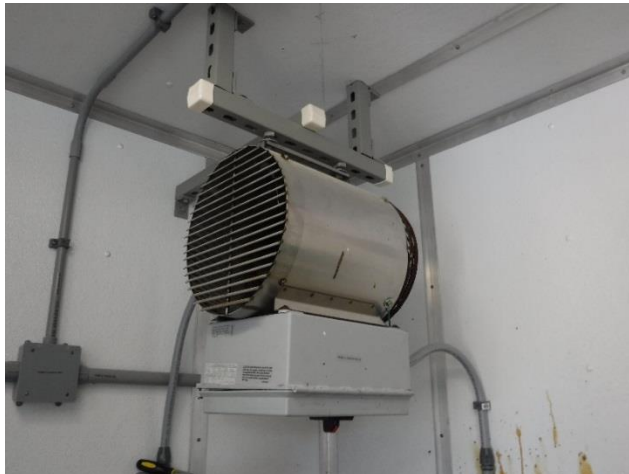
Figure 5: Chemical Room Electric Heater
