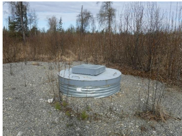
Figure 2: Tyonek Water Treatment Plant Well 2
