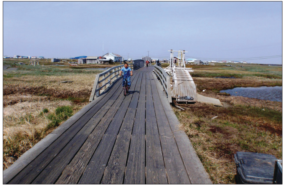
Boardwalks are an important part of the community infrastructure in Kwigillingok. DEHE FILE PHOTO
