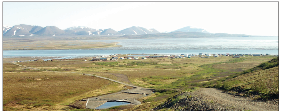
Goodnews Bay received water and sewer services for the first time this past year. DEHE FILE PHOTO
