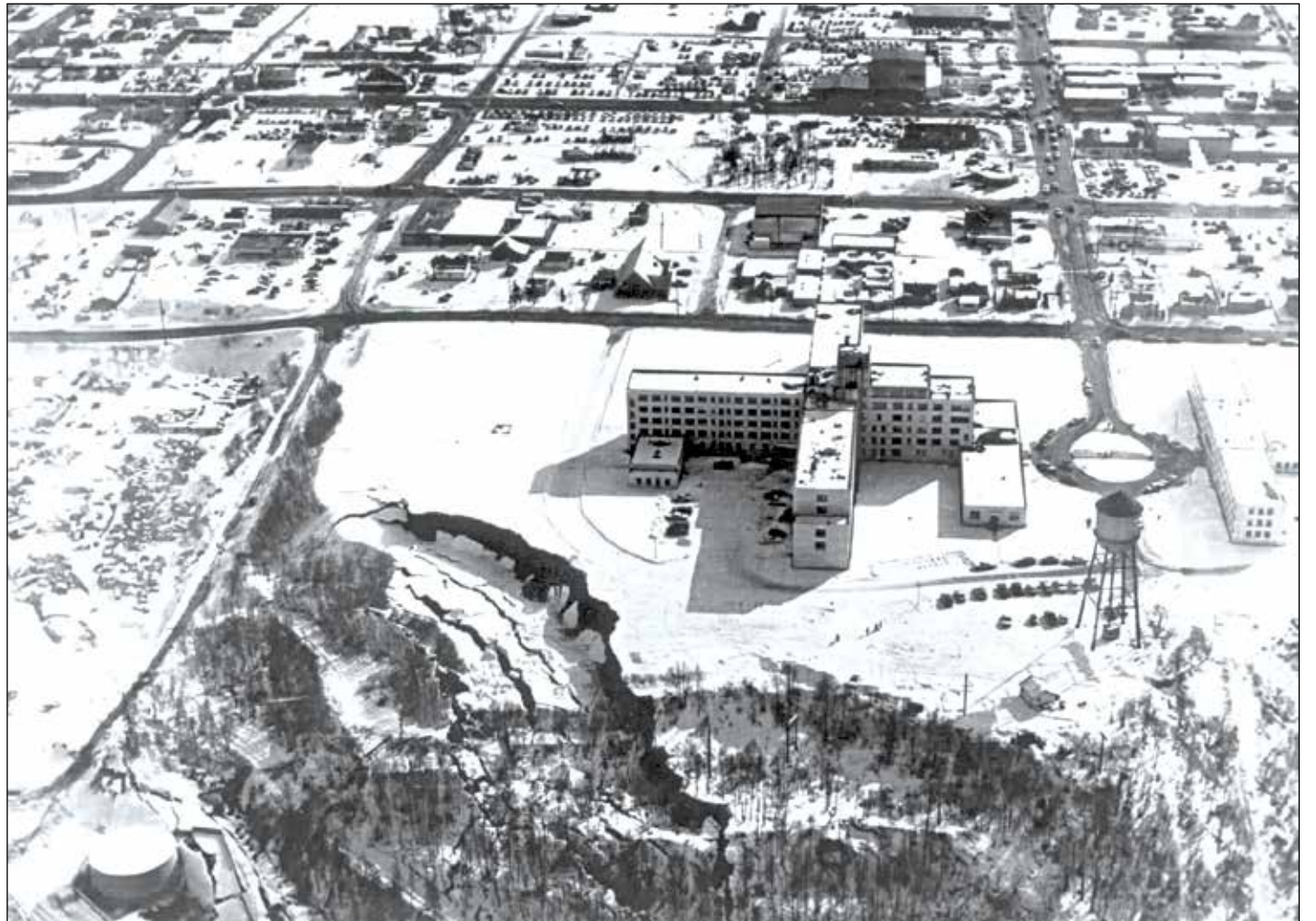
The original Anchorage Medical Center of the Alaska Native Service narrowly avoided a landslide and catastrophe during the Good Friday Earthquake of 1964.
