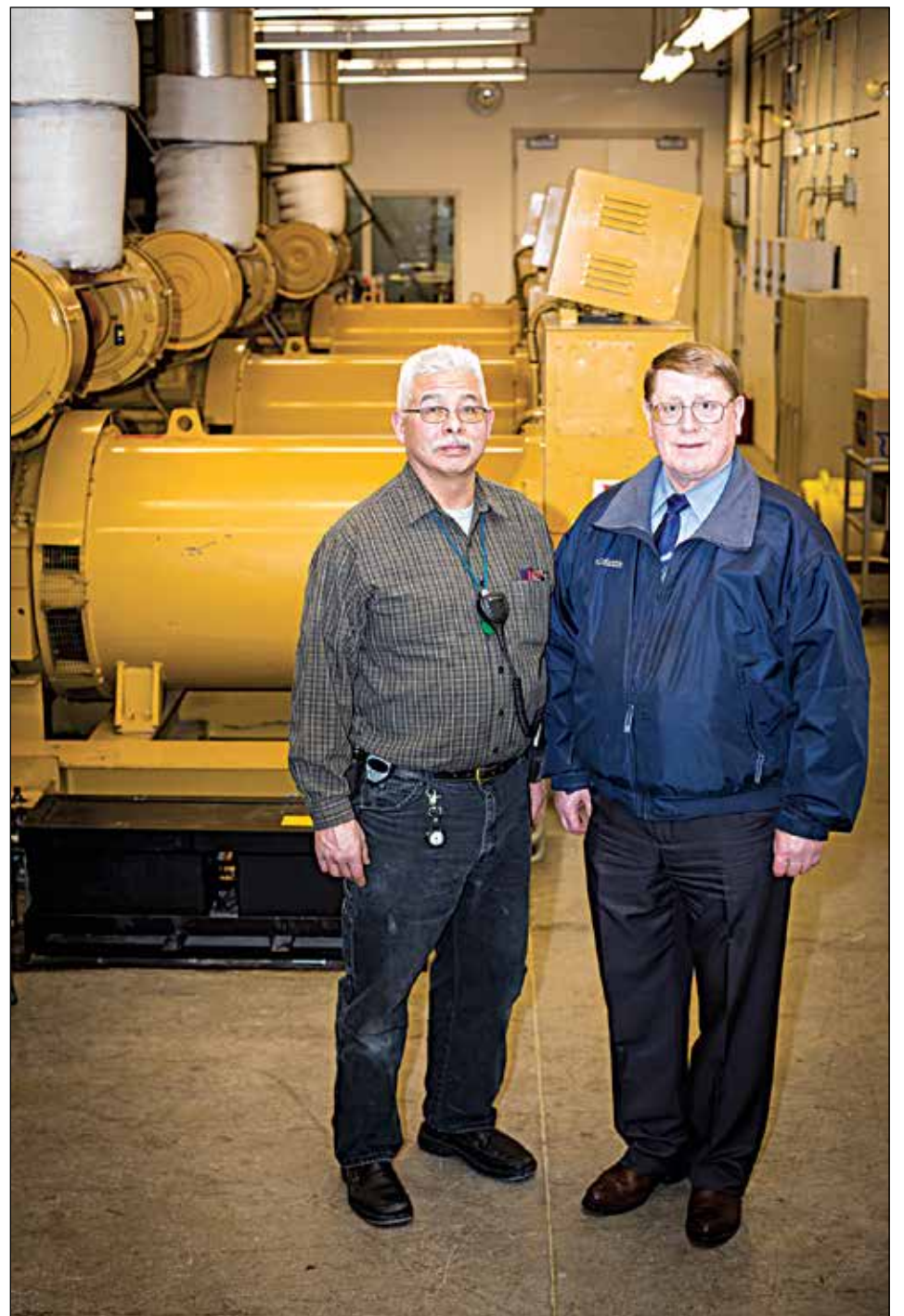
PHOTO BY TODD HENRY / ANTHC Supervisor of Facilities Mark Roehl, left, and Director of Facilities Services Robert Wilson show off the backup generator room in the basement of the ANMC hospital.
