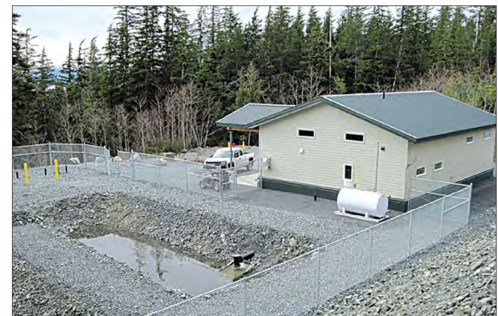
PHOTO BY JERRY CNOSSEN / ANTHC The new ANTHC-built, 1,500-square-foot water treatment plant in Kasaan opened this spring and is providing clean water to the area's residents.
