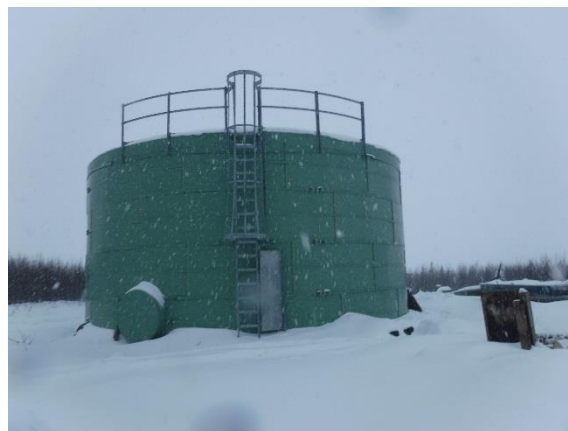
Figure 1: The Koliganek Water Storage Tank
