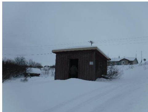
Figure 3: The Koliganek Lift Station
