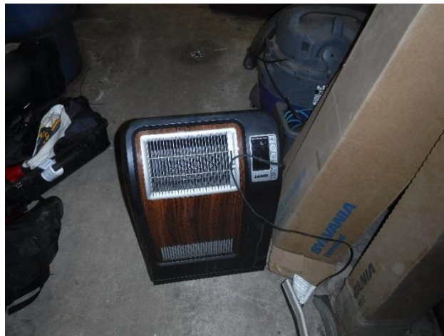
Figure 5: Portable Electric Heater in the Circle Washeteria
