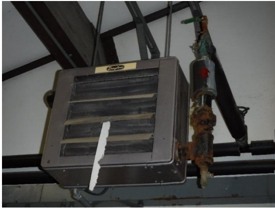
Figure 6: Broken Unit Heaters in the Circle Washeteria
