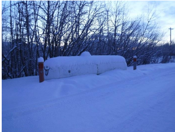
Figure 4: Propane Tank outside the Circle Washeteria
