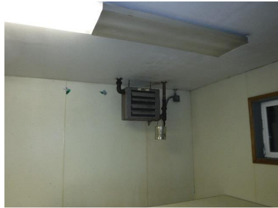
Figure 6: Broken Unit Heaters in the Circle Washeteria
