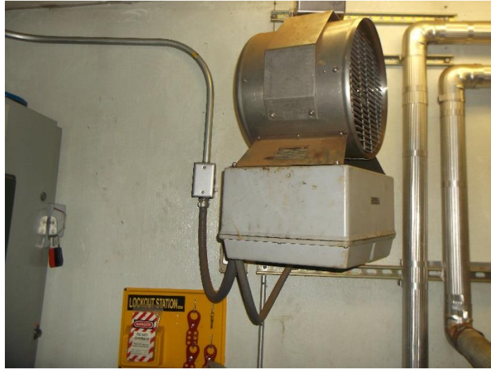
Figure 3.2: Electric Space Heater in the Pump House
