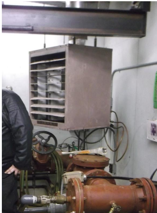
Figure 3.1: Fuel Oil-fired Unit Heater in the Pump House
