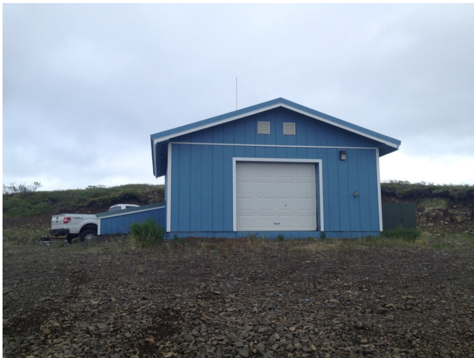
Sand Point Water Intake Facility
