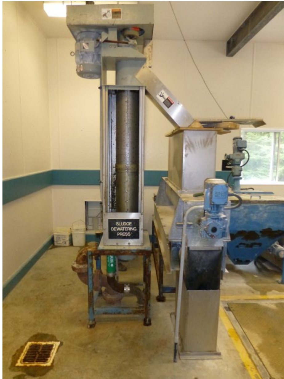
Figure 5: Sludge Dewatering Press
