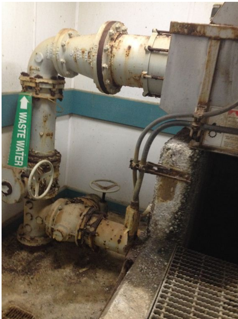
Figure 2: Inlet Piping and Concrete Damage
