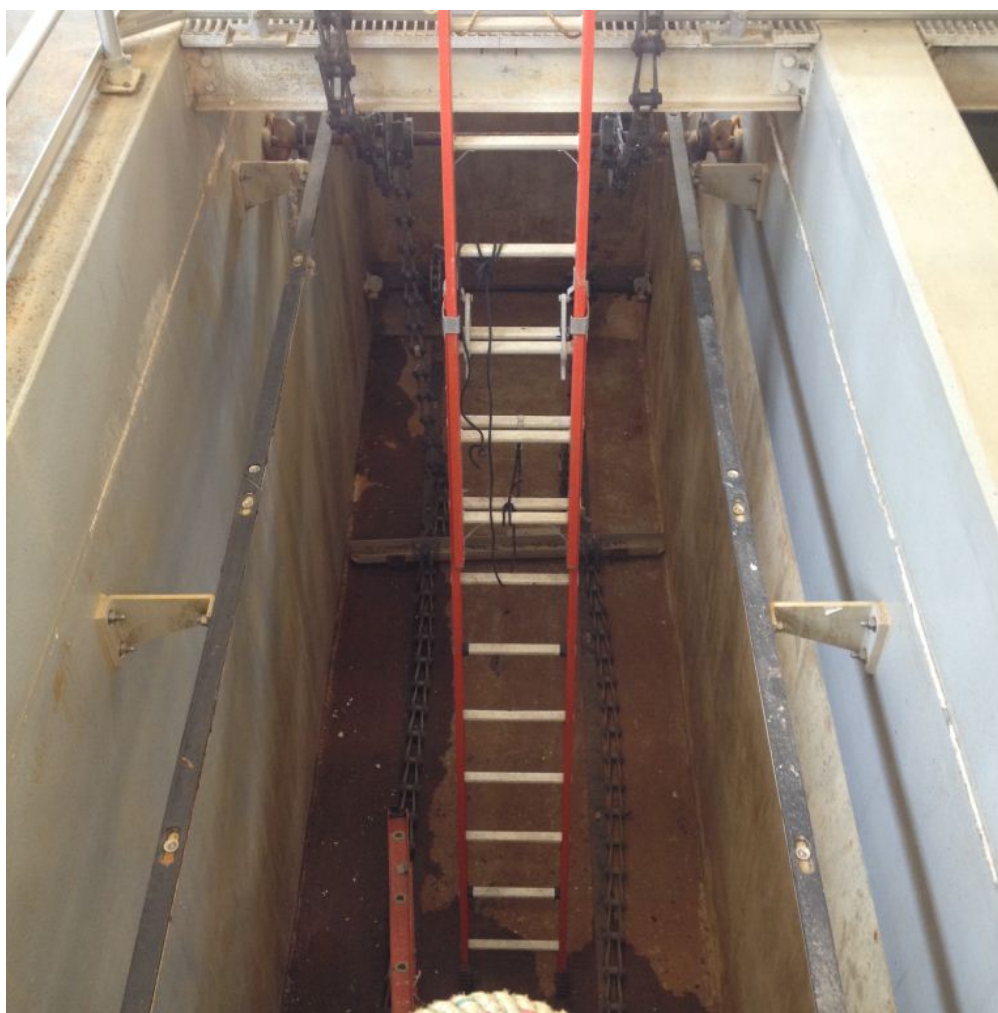
Figure 6: Primary Clarifier Skimmers and Scrappers
