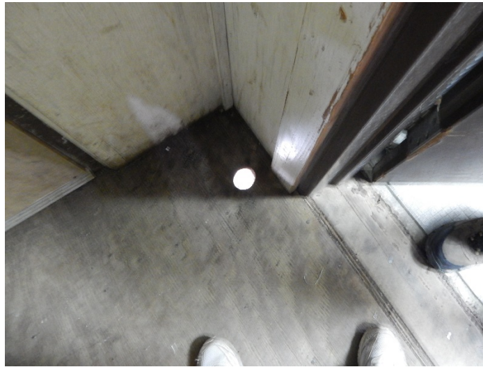
Figure 1: Hole in floor of the arctic entry that needs to be repaired.
