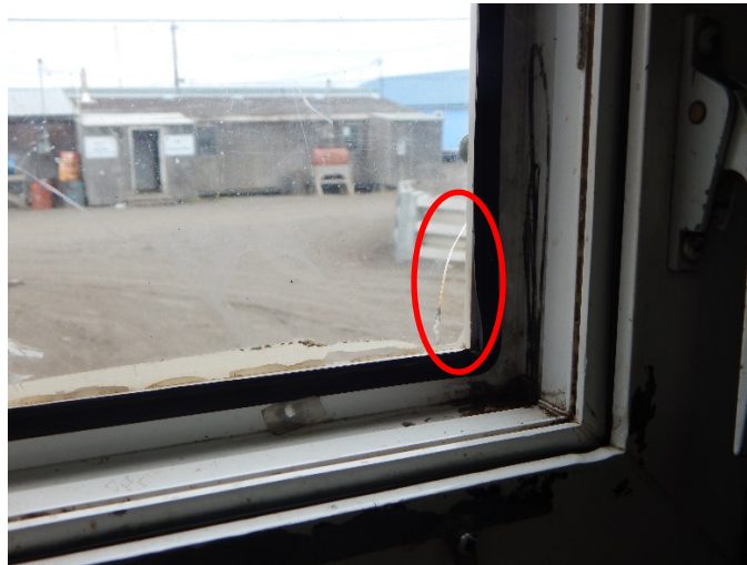
Figure 2: Broken Window that needs to be replaced, located in the mechanical room, north wall.
