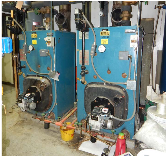
Figure 5: Burnham V-904 boilers in the WTP.
