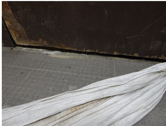
Figure 4: Door leading to the washeteria with a visible gap where air tightening and weatherization needs to be implemented.
