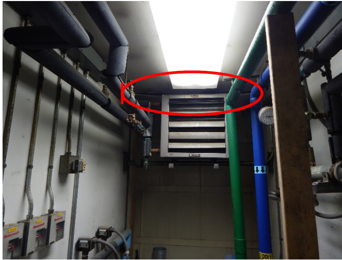
Figure 6: Unit Heater next to the treated water storage tank, coming off of its fixtures.
