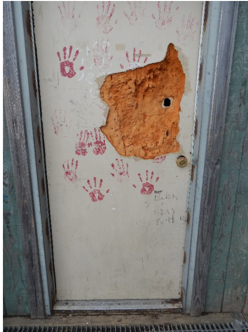
Figure 3: Damaged door leading to the arctic entry that needs to be replaced.
