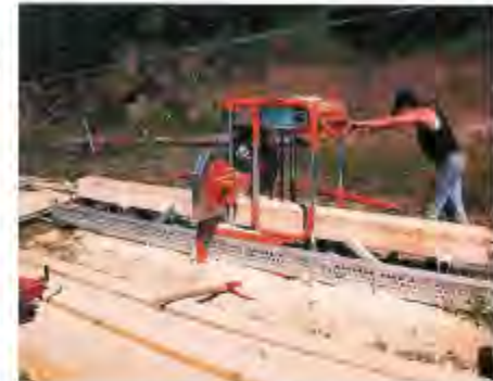
Milling lumber for the Napaimute storage building
