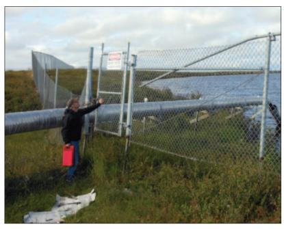
Sinking and erosion has damaged the sewage pond outfall.
