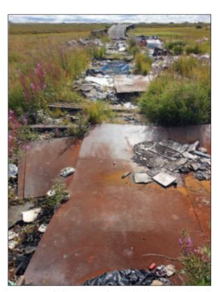
A damage section of the dump board road. Raj Chavan, 2011.
