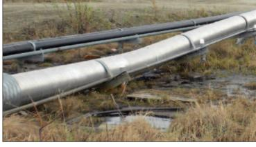
Arctic pipes, sagging as they sink into the ground.
