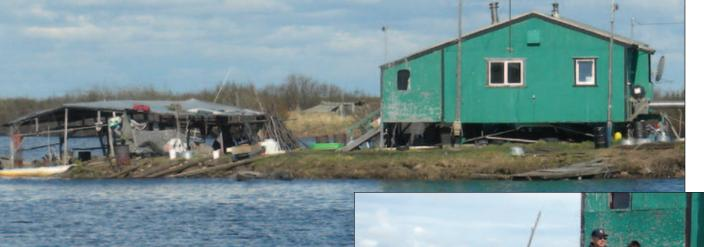
2. The riverbanks are eroding causing loss of property and threatening homes. An estimated 36 homes in Selawik are vulnerable to bank erosion, with some areas losing several feet of riverbank each year. Erosion prevention has been used successfully in the past and should be reconsidered for the future based on a bank soils study. Without immediate mitigation measures some houses will need to be moved before they flood
