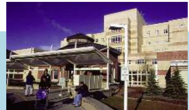
Completes several hospital remodeling projects, including the day-surgery area, the addition of an operating room, and renovation of the laboratory, and expanded guest areas in Quyana House.
