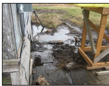
Old, exposed area now protected
