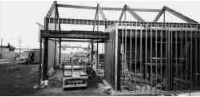
Top: The New Emergency Room addition for Kakanak Hospital in Dillingham was one of 37 projects built by the Division of Health Facilities. Bottom: the addition under construction.
