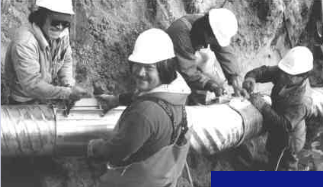
South Naknek workers connecting Fred Kraun's house to main sewer lines. Left to right: Hank Agwiak, Martin Angasan, Unidentified, Mike Johnson.
