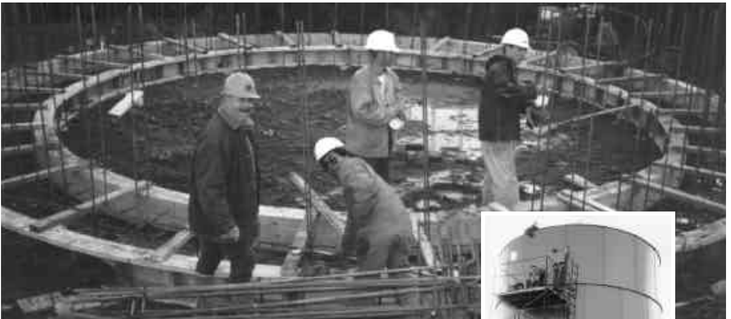
South Naknek workers forming the concrete-ring wall foundation for a 100,000 gallon bolted steel insulated water storage tank. Left to right: Milt Hanson, Mike Johnson, two unidentified workers.
