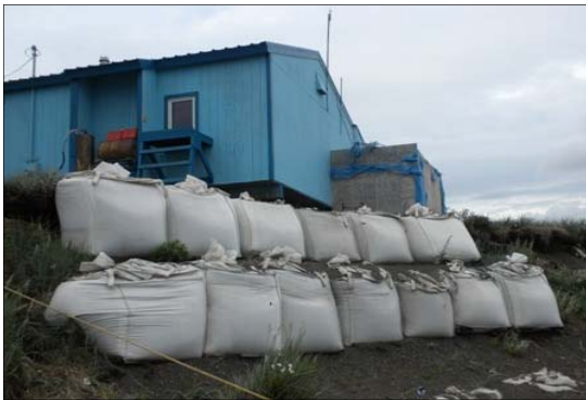
Erosion damage to a home in Kivalina Photo Courtesy Mike Brubaker
