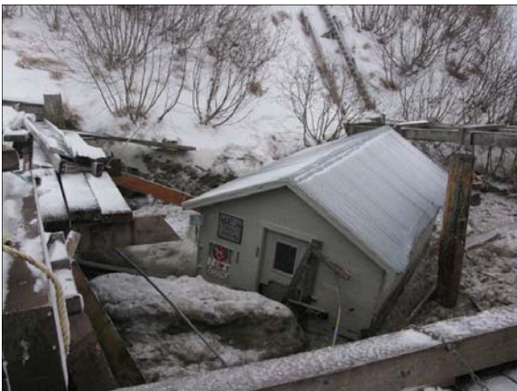
Flood damage in Naknek Photo Courtesy John Warren
