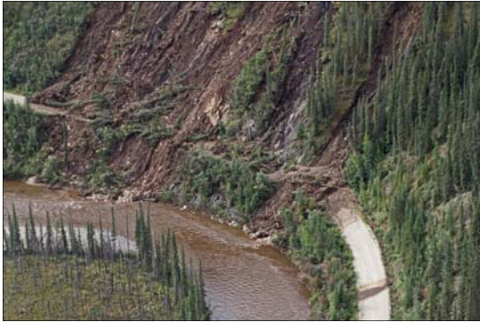
Landslide on the Taylor Highway Photo Courtesy of DOT 2010
