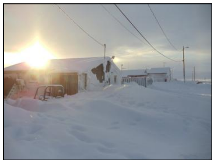
Ice storm in Savoonga resulted in power outages and loss of water service Photo Courtesy ADN
