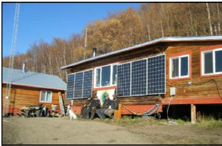
In the fall of 2010, the Native Village of Napaimute installed solar panels and a small wind turbine to provide year-round power to their tribal office Photo Courtesy Mark Leary
