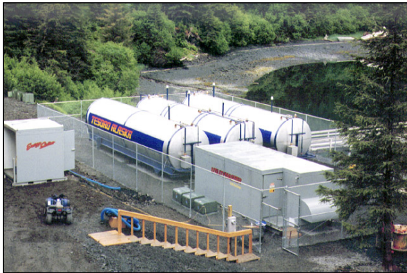
An upgraded tank farm with secondary containment Photo Courtesy Bill Stokes
