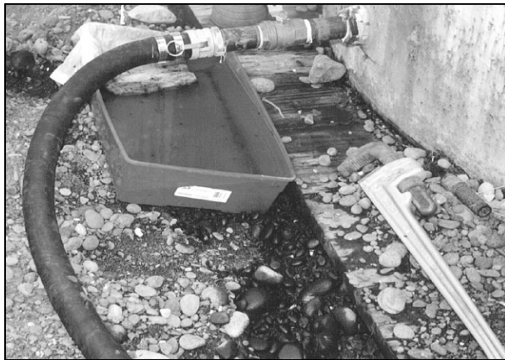
Even small leaks turn into large fuel spill over time
