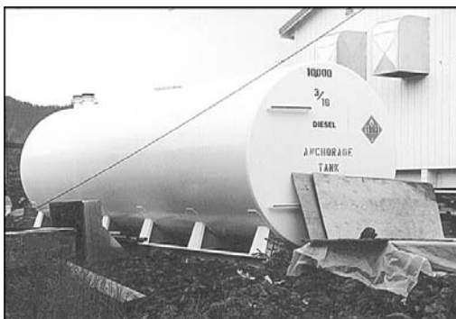
All tank farms should have clear and visible labels identifying the contents inside
