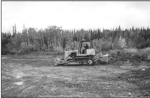
Bulldozer being used to consolidate, compact and cover waste at the landfill
