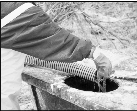
Flush-haul operators may be exposed to raw sewage when emptying the tank Photo Courtesy Joe Sarcone
