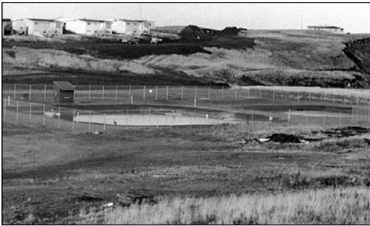
Sewage lagoon located below the residential area of a village
