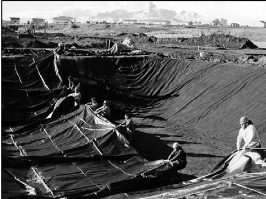
Building a sewage lagoon with a liner Photo Courtesy Kurt Egelhofer
