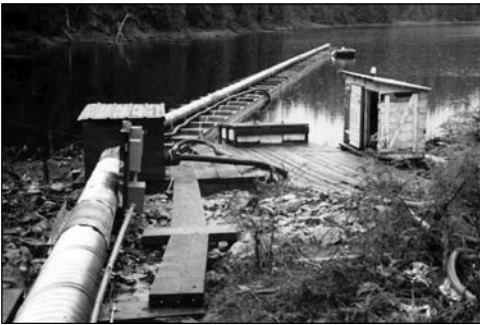
Surface water system Photo Courtesy Kurt Egelhofer
