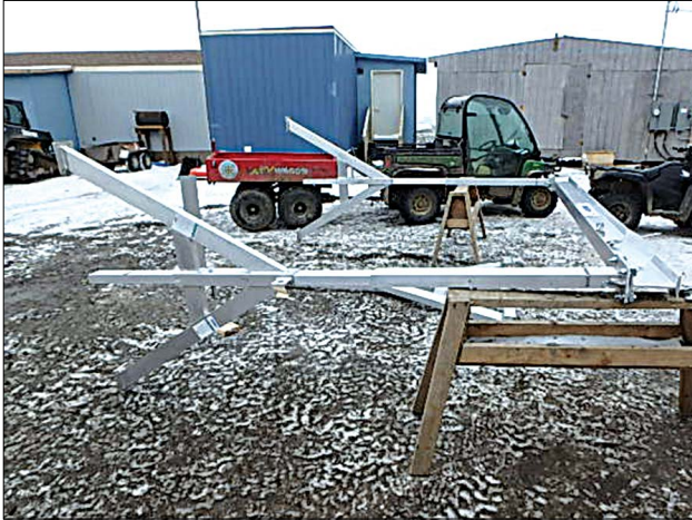
Above: Instead of operating a heavy excavator on the frozen river, Eek construction crews had to build a suspended crane system to support the water intake piping. Below: The ANTHC Environmental Health and Engineering team came together to find a solution for year-round access to clean water in Eek.
