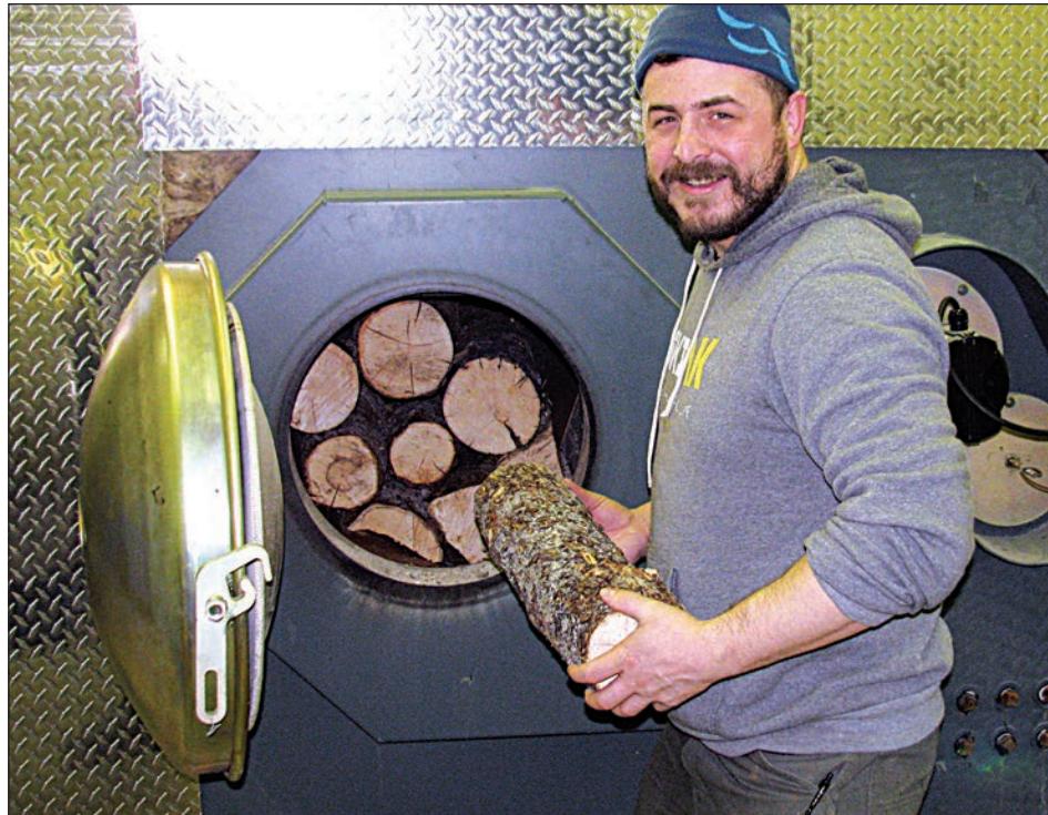
Kyle Monti, Utility Operations Specialist, loads the new Kobuk wood heating system.
