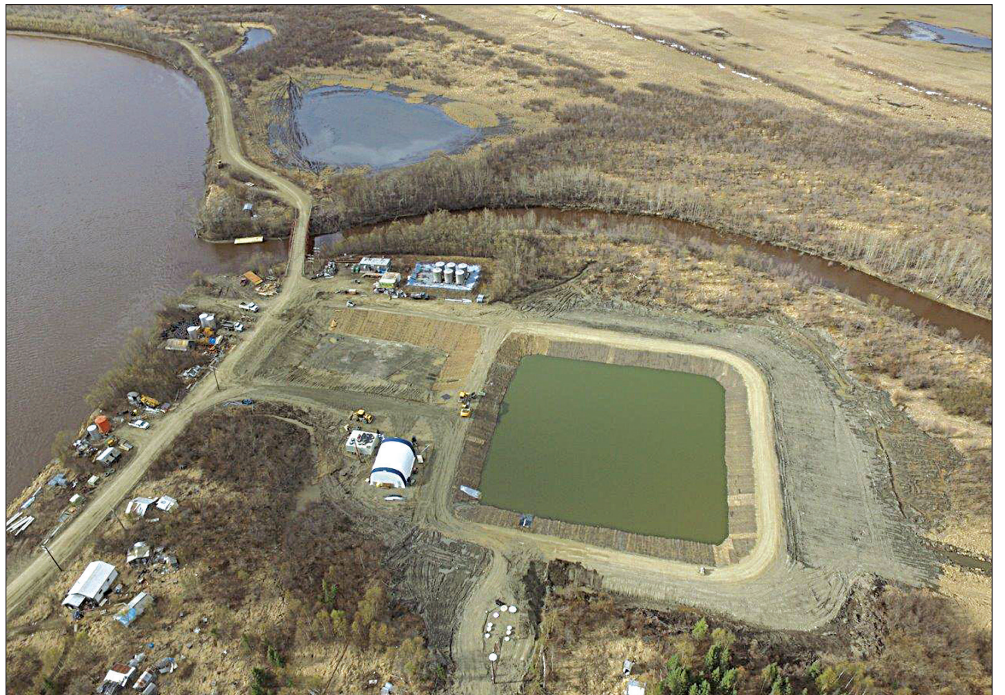
Above and below: New wastewater lagoon in Shageluk.
